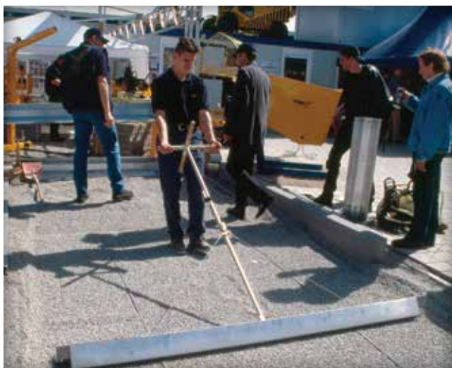
Figure 24. Manually screeding the No. 8 stone setting bed.
