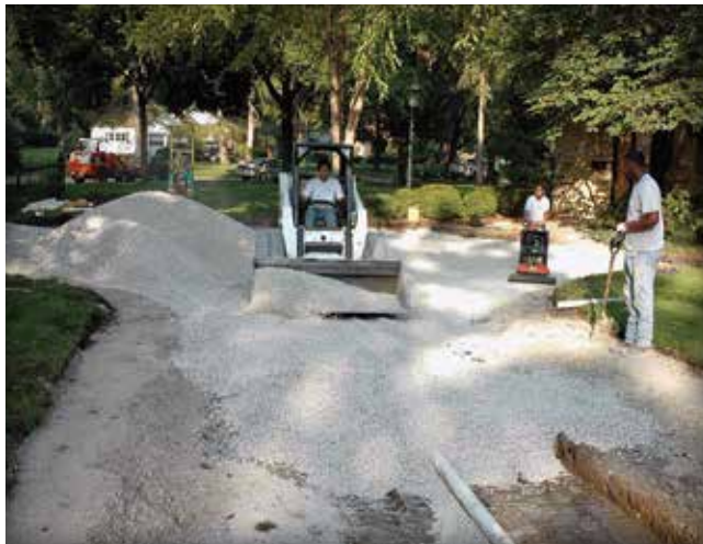
Figure 17. Perimeter berms made with dense-graded base are in place prior to placing open-graded aggregate in the driveway.
