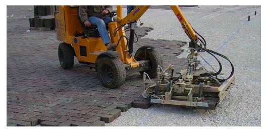
Figure 5. Mechanical installation of concrete paving units for PICP.
