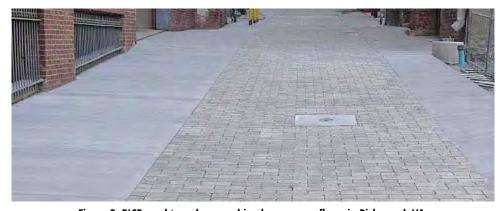
Figure 3. PICP used to reduce combined sewer overflows in Richmond, VA.
