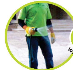
LIGHT MIST TO LOCK THE JOINT
