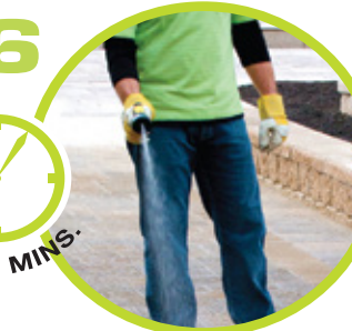
HEAVY SPRAY TO CLEAN THE PAVERS
