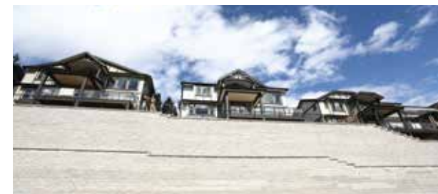
Large Retaining Wall Projects
