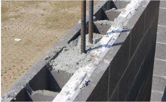
Figure 7a – prior to joint reinforcement
