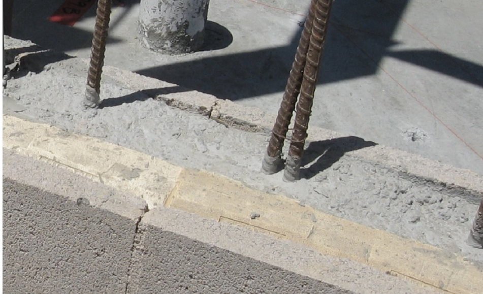
Figure 2 – Reinforcement centered in grouted area of 12 inch Hi-R H
