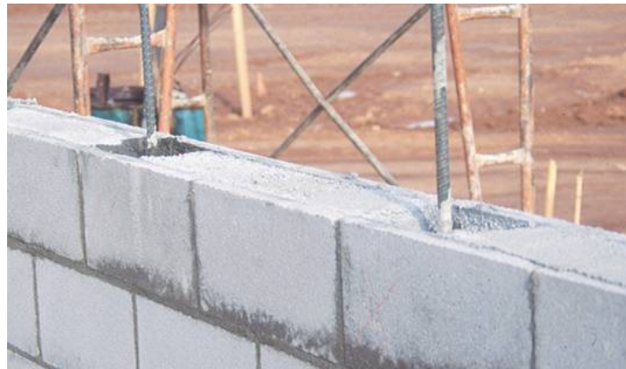
Figure 1- Conventional reinforced masonry with reinforcement in center
